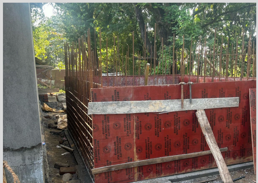
Advancement of RCC Storage Tank construction in Mothapara village. Also, the formwork for an RCC water tank is currently underway in Abendagre village.
